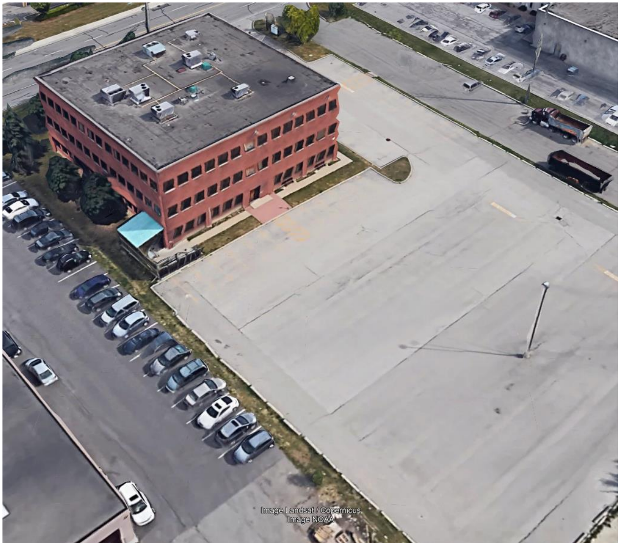
Figure 3 : Aerial View Rear of Building
