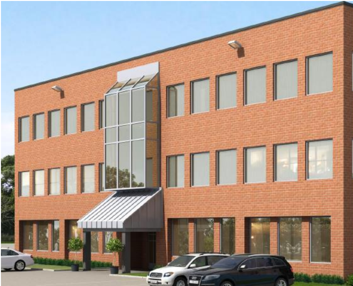
Figure 2 : East Entrance Face of building
